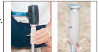
**3.** Remove the Driver and insert the AccuScreed Yoke into the conduit. Regardless of the angle of cut or the degree of rotation, the Yoke will maintain the exact position as indicated by the height marker. Repeat this same procedure for each screed location.
