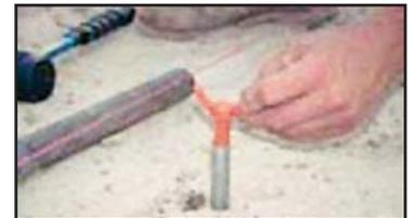
**4.** Set the 1-5/8" O.D. Screed pipe on top of the Yoke and you are ready to pour. The top of the screed pipe will precisely match the strike off point! The conduit, which fills with subgrade and concrete, remains in place. AccuScreed Yokes are cost effective and will not expand, allowing the contractor to leave them in the pour. It's simple, fast and convenient!
