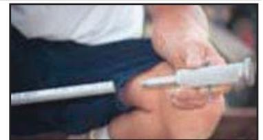
**2.** Insert the AccuScreed Driver into the conduit. Using the AccuScreed Dead Blow Hammer, strike the top of the Dead Blow Hammer, strike the top of the Driver unit the height marker aligns with the string line or laser.
